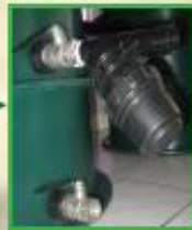
Outlet Tap 32mm Drain fitting 32mm Outlet sedimentation filter (Optional)
